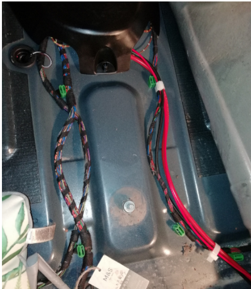
Above: shows the front cab under rubber floor wiring routes, alongside the VW standard wiring
