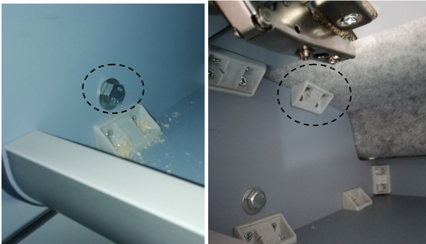
Above: Top 'above bed unit' showing bolt to rear furniture & left hand top fixing to the ply above
