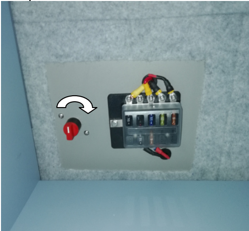
Isolator switch and fuses, the isolator turns Clockwise to turn On (off position shown)
