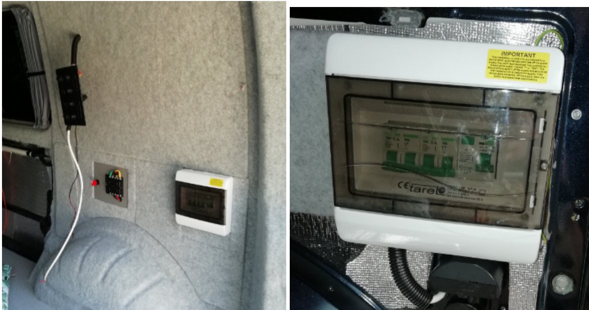
This shows the arrangement of the main electric systems behind the furniture on the OS rear of the van, the hanging switch panel screws into the rear furniture. The right pic shows the connection to the hook up point.
