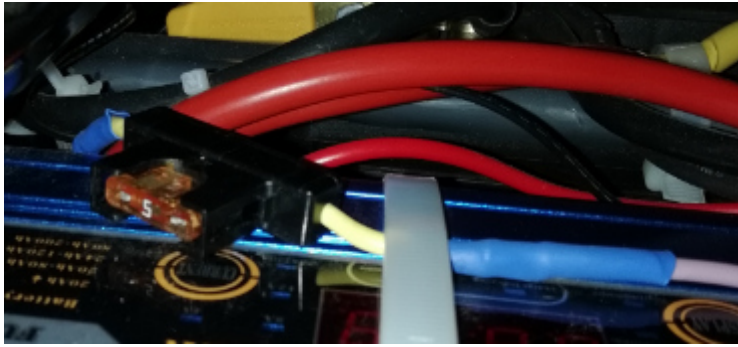
Above: Fuse (5A) supplying the voltage display for the Van Battery
